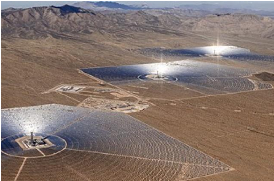
Cea mai mare instalație termoergetică cu turnuri solare Ivanpah Solar Power Facility, USA (San Bernardino County, California – 392 MW) http://www.iflscience.com/sites/www.iflscience.com/files/styles/ifls_large/public/blog/%5Bnid%5D/80_630_225_stillings1.jpg?itok=xTGJSu3i
