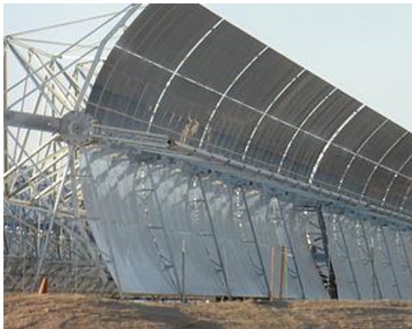
Colector solari termici cu concentratori parabolici (Harper Lake, California, USA) https://en.wikipedia.org/wiki/File:Parabolic_trough_at_Harper_Lake_in_California.jpg
