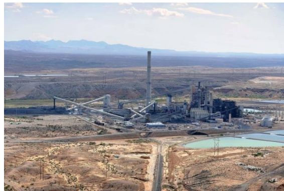
Imagine a centralei energetice Reid Gardner
